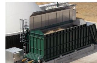
The digester is filled with solid resources by means of the Thöni loading system for solid matter. From there, the quantities are fully-automatically metered into the digester
